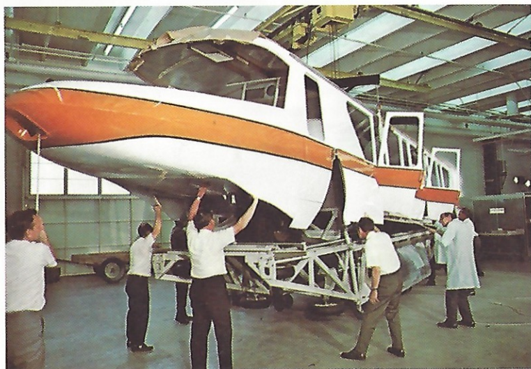
VISITOR TRANSPORTATION: Two 200-passenger sidewheel steamboats, three narrow-gauge steam trains and six 212-passenger monorail trains are being readied to serve Walt Disney World visitors on opening day. The silent, all-electric monorail trains will travel atop three-and-one-half miles of twin-rail concrete beamways, soaring as high as 60 feet above the ground. 337 monorail beams, each 85 to 110 feet in length, are being cast in Tacoma, Washington, and shipped to the site by rail.
