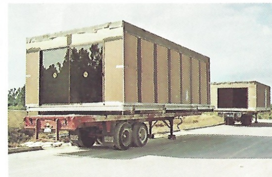
MODULAR CONSTRUCTION: The first two hotels at Walt Disney World will feature guest rooms of lightweight modular steel construction. Fabricated in an on-site assembly plant (left), the rooms are trucked to the construction area, where they are lifted into place and utilities are plugged in.
